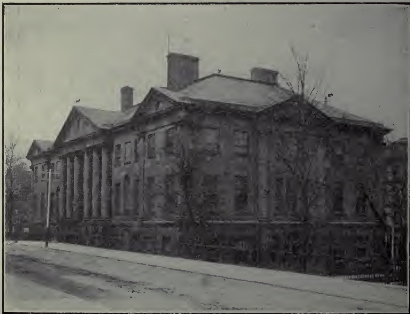
PROVINCE BUILDING, HALIFAX.
